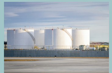
Tank to Tank
